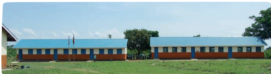
The new classroom blocks at Orapwoyo.
